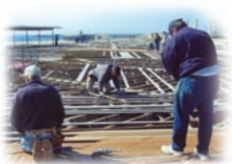
The new planks are fastened in place.
