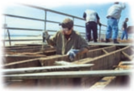
All planks on the half-mile boardwalk had to be removed.
